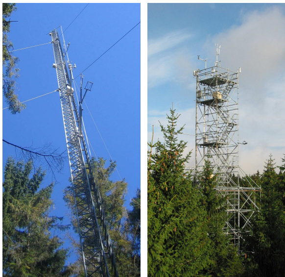
Figure 1: The 36-m turbulence tower (left) and the 32-m main tower (right) at the Waldstein site.
