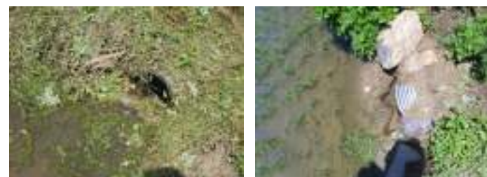
Fig. 2: Water drains without protective measures
