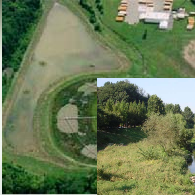
Olentangy constructed wetland
