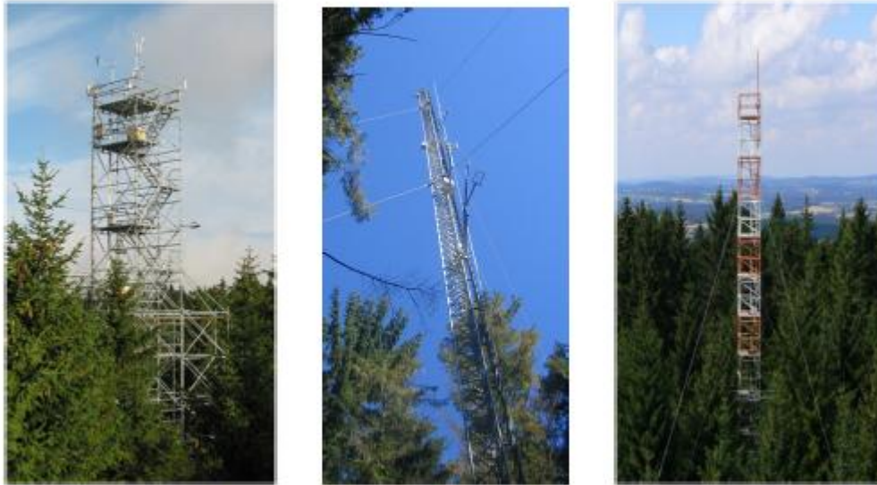
Figure S1. Towers at the Waldstein-Weidenbrunnen site: left: Permanent main tower since 1996 (height 31 m) for routine measurements, FLUXNET station and chemical measurements, middle: turbulence tower (height 35 m) since 2007 with second FLUXNET complex and turbulence measurements, right: biological tower (height 36 m) for gas exchange measurements at needles.
