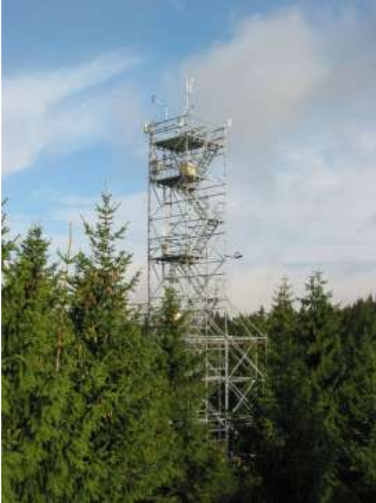
Figure 20. FLUXNET site DE-Bay (Waldstein-Weidenbrunnen, Bayreuth, Germany), Main tower for eddy-covariance and additional micrometeorological measurements.
